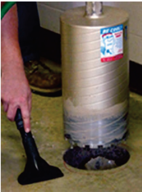
Figure 2.65 Concrete coring
