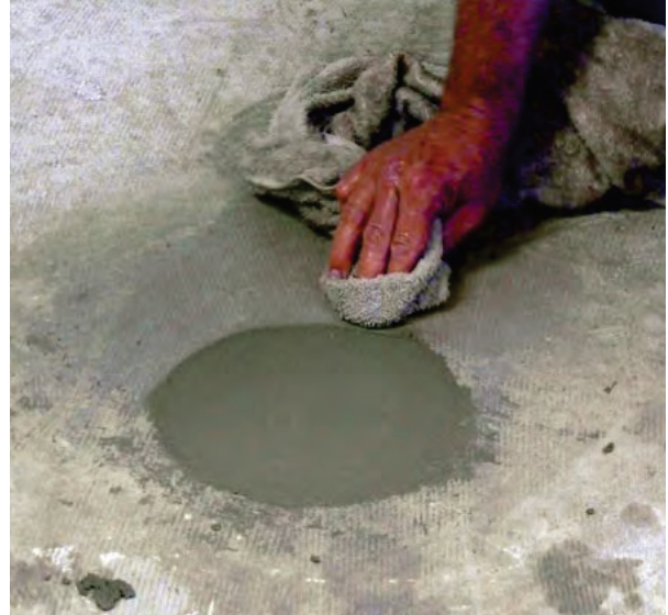
Figure 2.83 Finishing concrete
