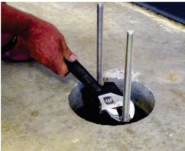
Figure 2.75 Lightly tighten pier cap down onto pier tube
