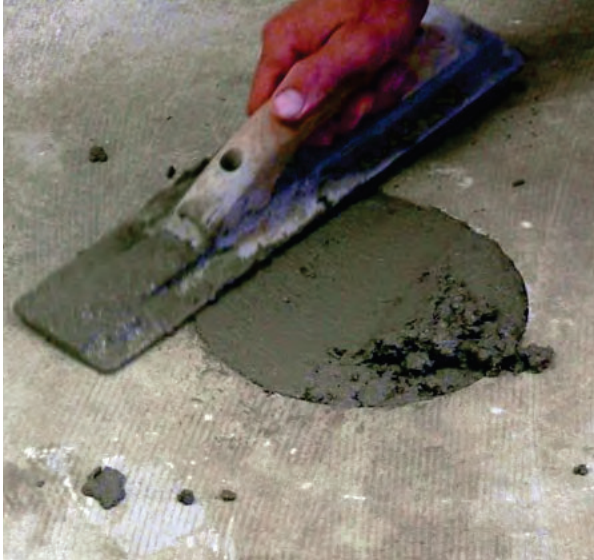
Figure 2.82 Patching holes at pier locations
