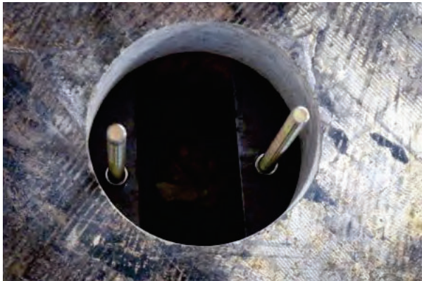
Figure 2.69 Threaded rods installed
