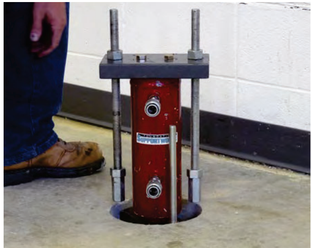
Figure 2.76 Lift cylinder assembly set on pier cap
