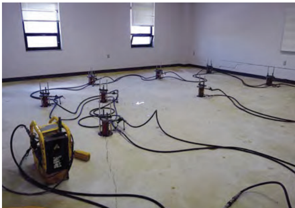
Figure 2.79 Lift cylinders connected for simultaneous loading
